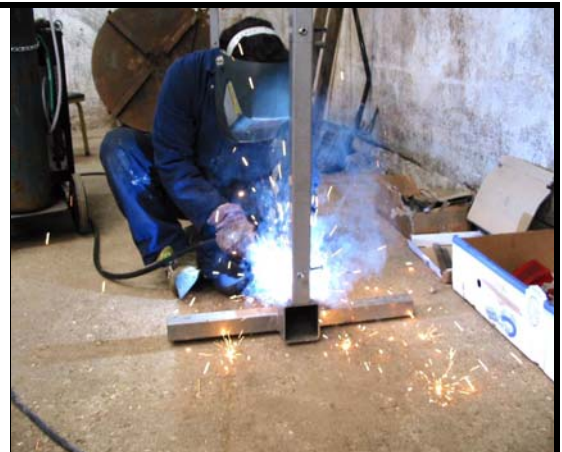
Mig welding at Carr's new factory in Kettering.
